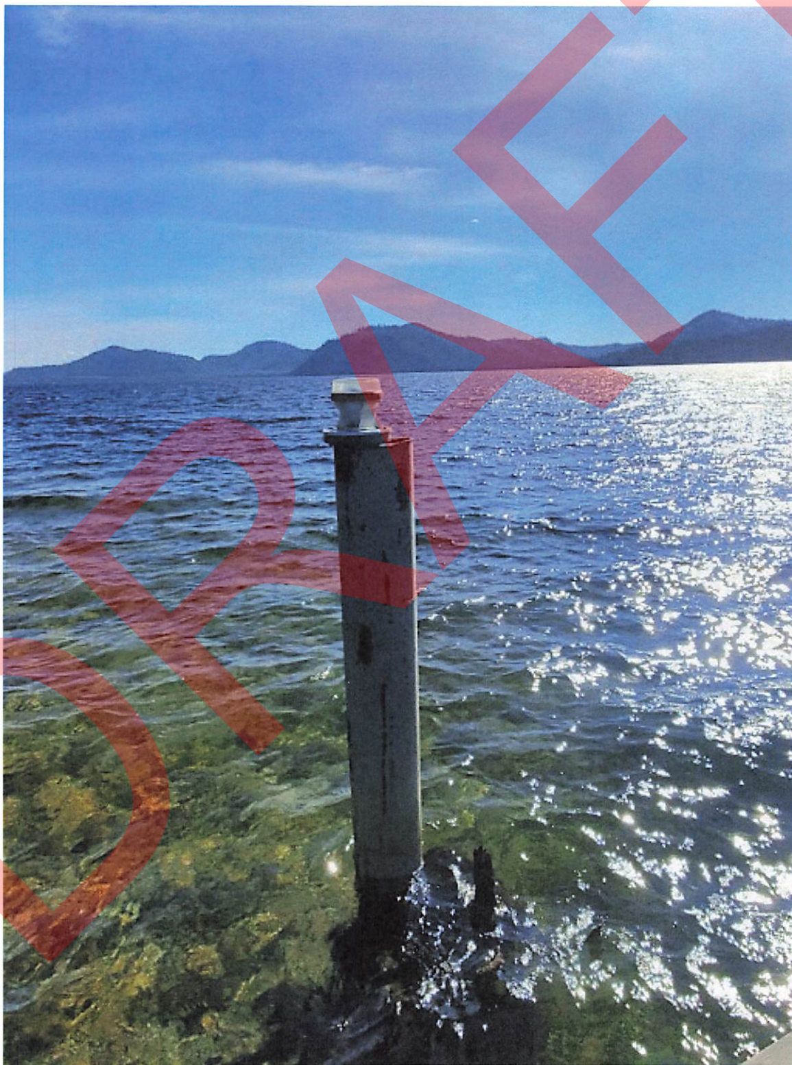
Pictured Below: New navigation light piling with new light
